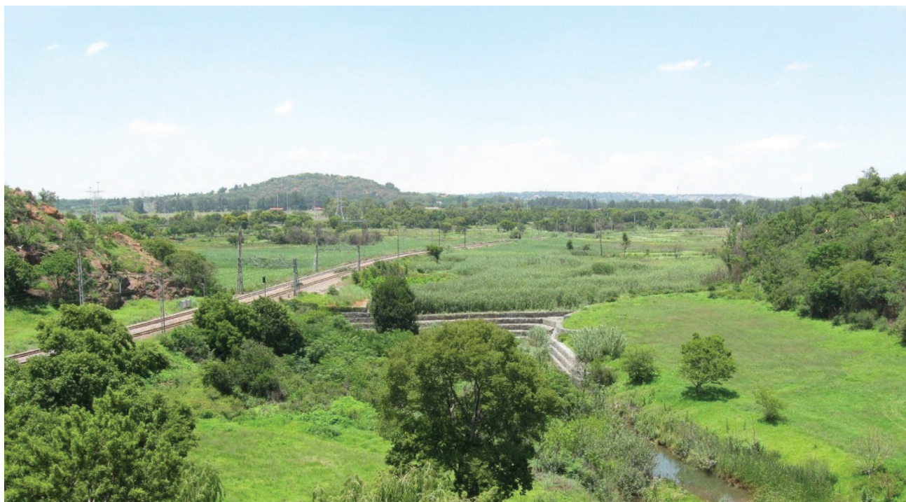
Figure 8: Gabion infrastructure constructed to control erosion in the Colbyn Valley Wetland
